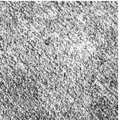
FIG. 5. - [PR] PERREADA // ROUGH-TROWELED - Acabado Picada con Ollos Profundos, Weathered Finish with Profound Holes
