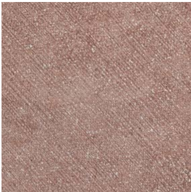
FIG. 5. [PR] PERREADA // ROUGH-TROWELED
