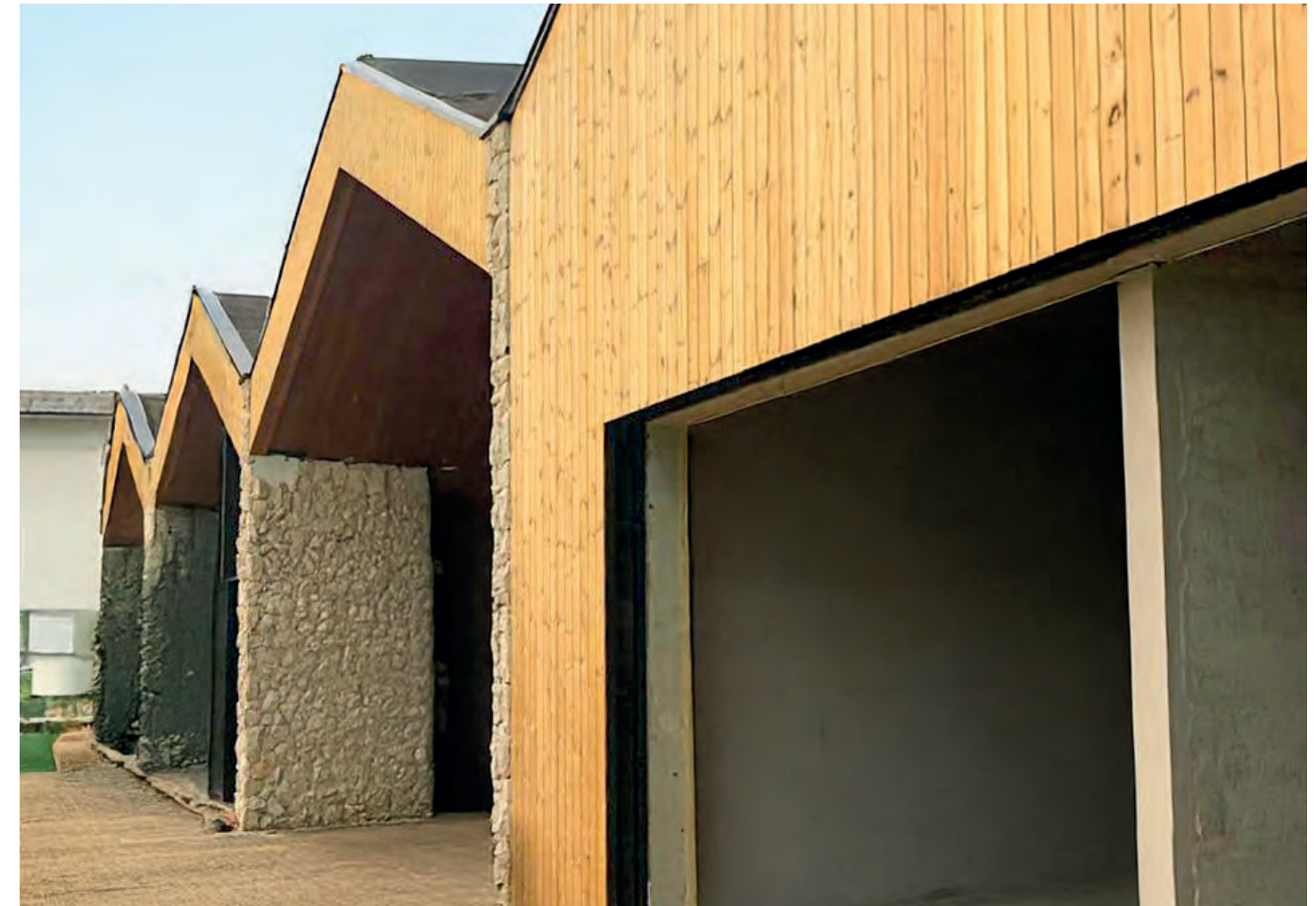
Scarsa Boutique, Thermowood W exterior, Arquitat, Colombia
